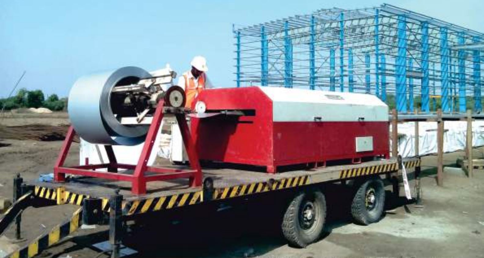
TRACDEK® SS-2000® On-site Roll Forming for Single Length Panels
