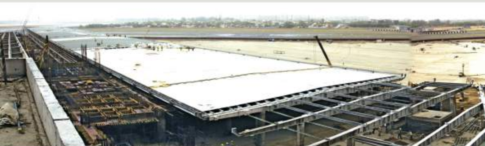
Pre-Engineered Structural Steel & Multi Layer Roofing Systems - IGI Airport Terminal 3 - Panoramic View International PIER Roof
