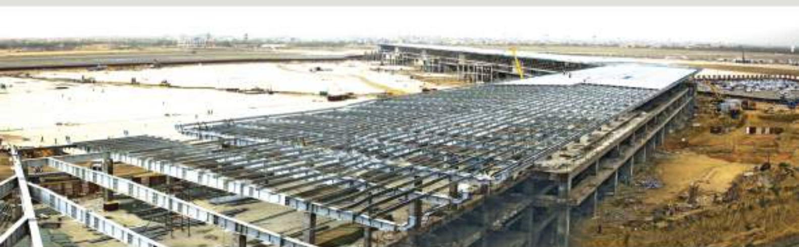
Pre-Engineered Structural Steel & Multi Layer Roofing Systems - IGI Airport Terminal 3 - Panoramic View International PIER Roof
